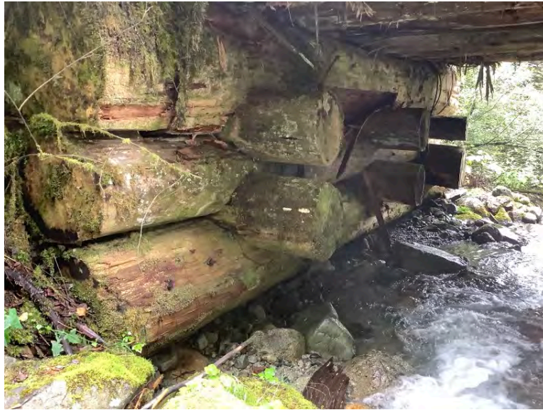
Left Bank Abutment when facing downstream
