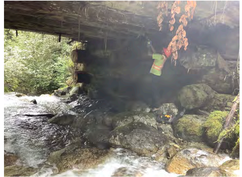
Right Bank Abutment when facing downstream
