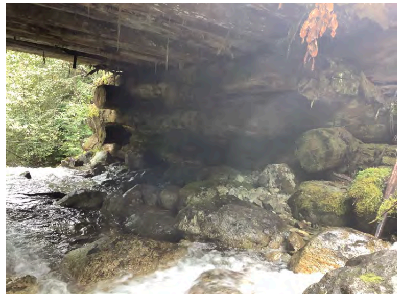
Right Bank Abutment when facing downstream
