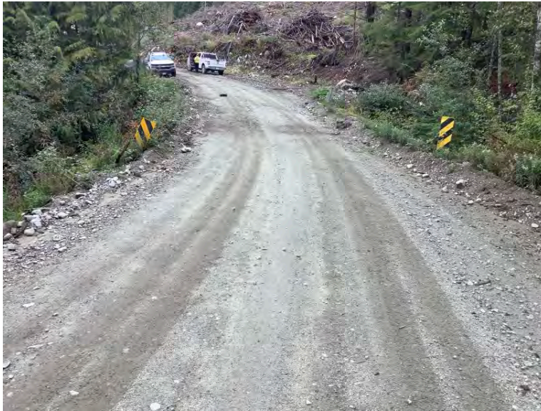
Left Bank Abutment when facing downstream
